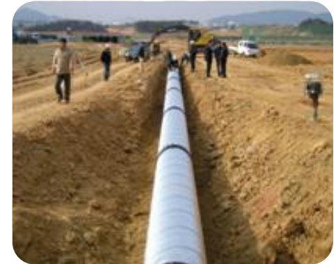
Installing CS Pipe
