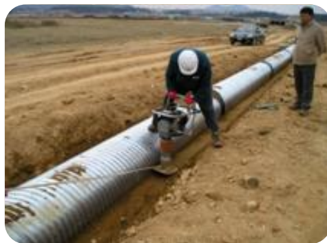
Backfilling
