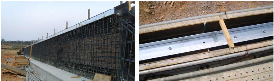
picture 2.1.1 Installing fixed channel
