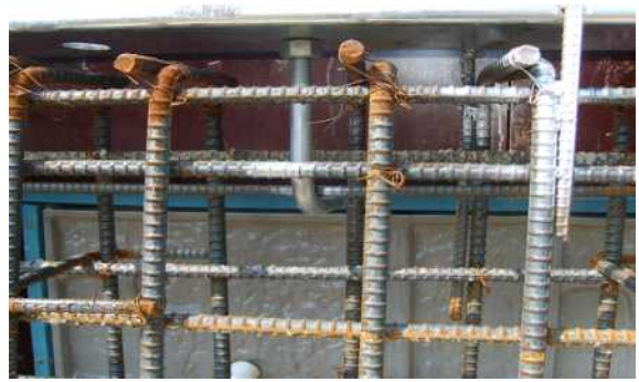
picture 2.1.3 Fixing L shape anchor
