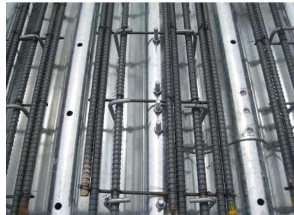
picture 4.1.2 rods after anchor installment.
