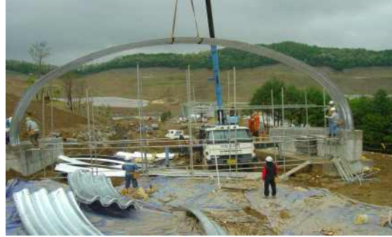
picture 2.2.3 connecting plates to channel
