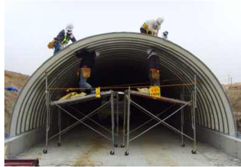
picture 2.2.6 construction of corrugated steel plate
