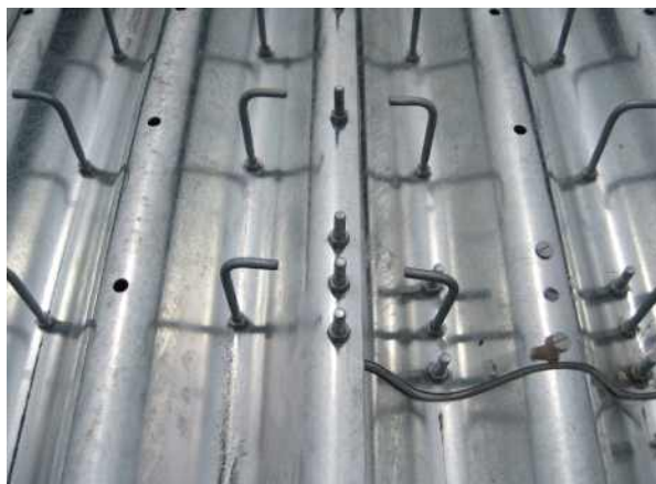
picture 4.1.1 CBS anchor installment
