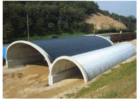
PE-SHEET water proof on upper side of CBS
