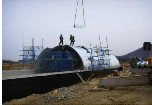
picture 2.2.6 construction of corrugated steel plate
