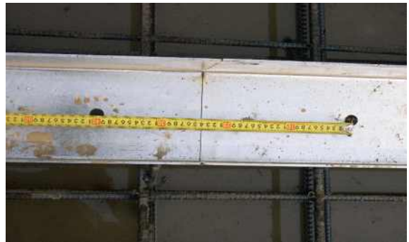
picture 2.1.5 distance of anchor hole
