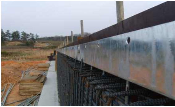
picture 2.1.2 Installing fixed channel
