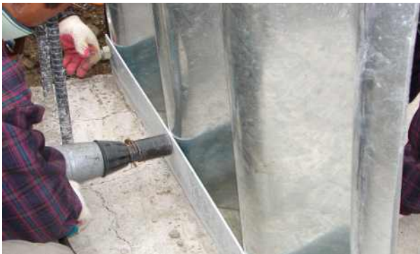
picture 2.2.4 conclusion of channel to plate
